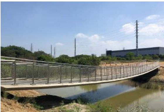
Straight pre-stressed hammock bridge structure
