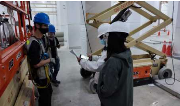
Manufacturing Industry/ TSMC Fab 18 New Construction Project (P7)
