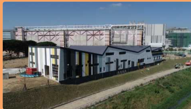
Distributing reservoir and Advanced treatment facilities
